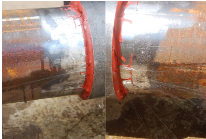
Figure 46: Leakages of specimen no. 4
