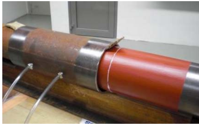
Figure 32: Aligned and surface pre-treated pipes, sleeve not centred
