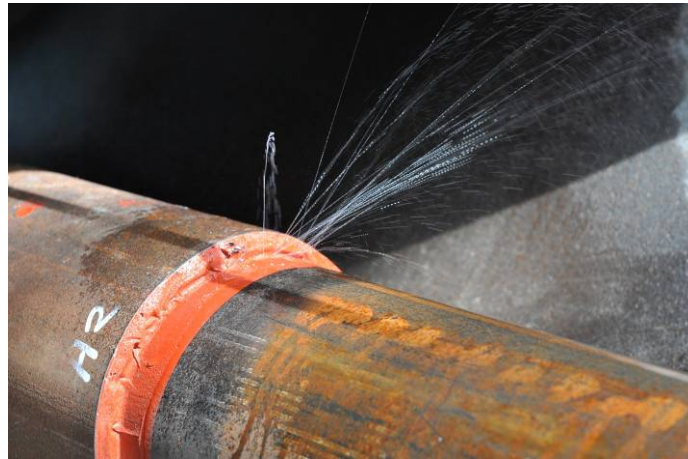
Figure 36: Leakage of specimen no. 1
