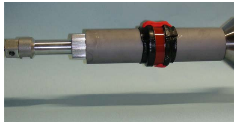
step 6c: injection complete, pipe joined
