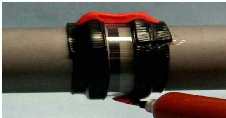
step 6b: filling of the gap
